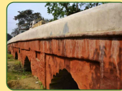
Namdang Stone Bridge
